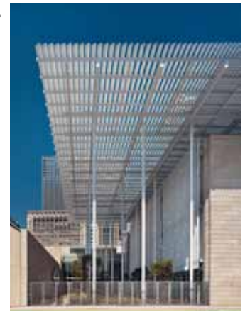
Figure 11 View looking east of the Modern Wing of the Art Institute, showing the "flying carpet" over the east portion of the building and the Turin and Agnelli Theater Gallery (see Fig. 10).
