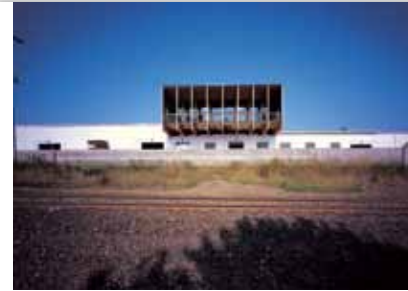
Above: The new office of the Hawks Boots Factory occupies an old factory building, illustrating a form of industrial building, illustrating a form of Duluth history.
